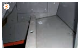
Main belt - wear protection
